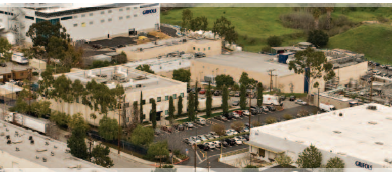
Grifols Fractionation Facility, Los Angeles, CA
