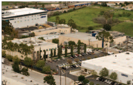
Grifols Fractionation Facility, Los Angeles, CA
