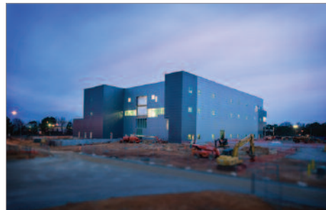
Grifols Fractionation Facility, Clayton, NC
