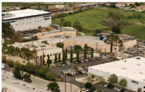
Grifols Fractionation Facility, Los Angeles, CA
